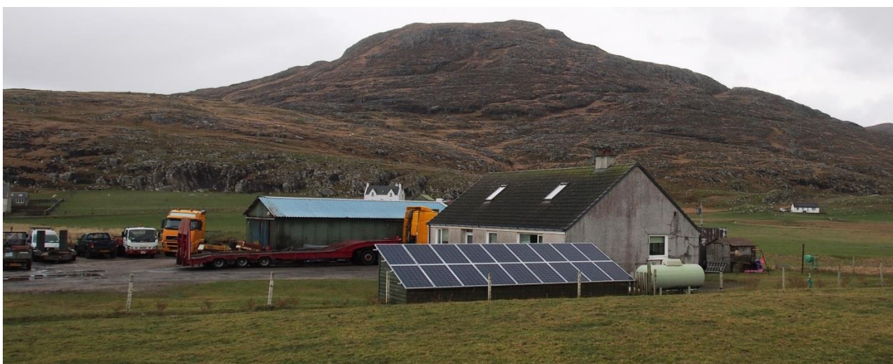
A business in Borgh on Barra uses a solar PV array to supply on site demand
