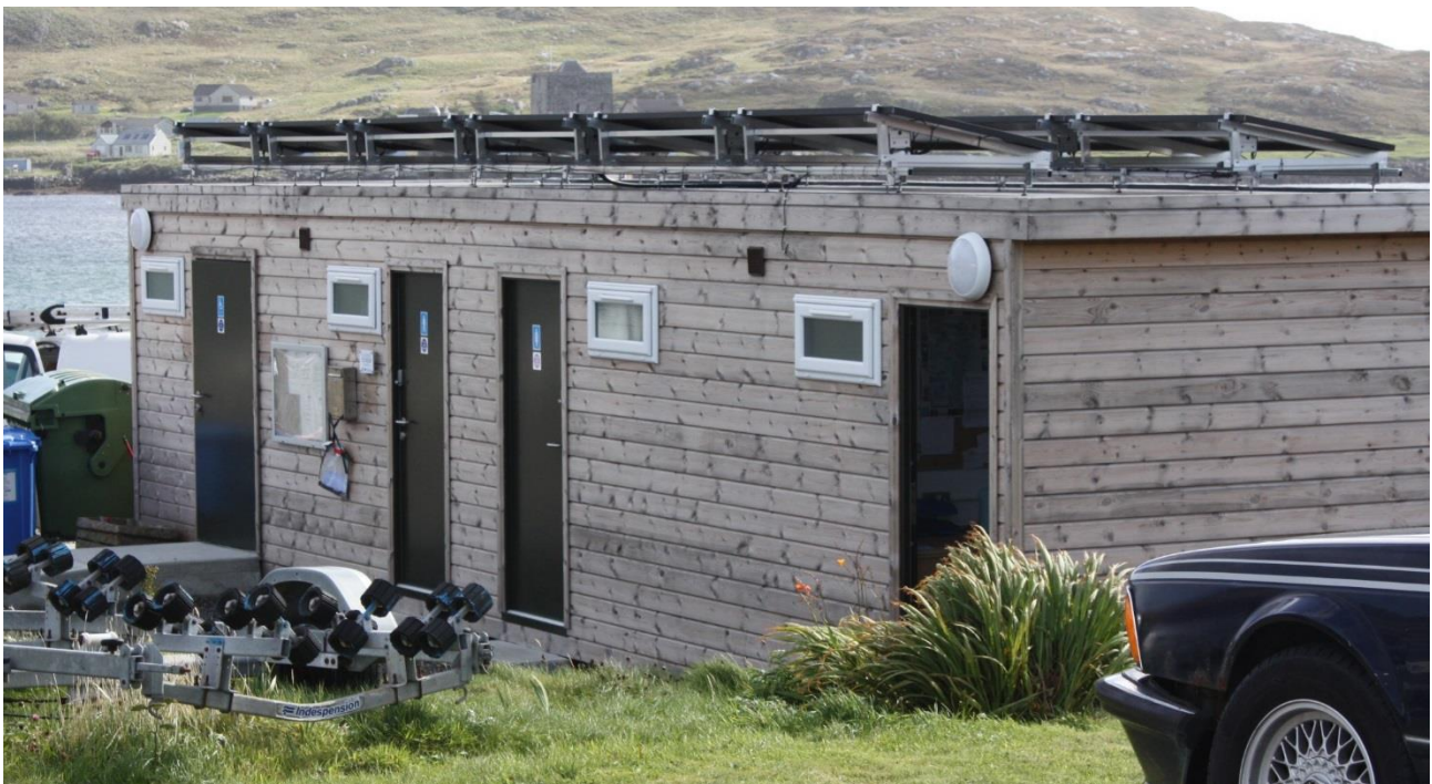
The shower and toilet block installed in 2019 at the pontoon in Castlebay, Barra, showcases a range of water saving and energy saving features and has a 4.2kW solar PV array on the roof.
