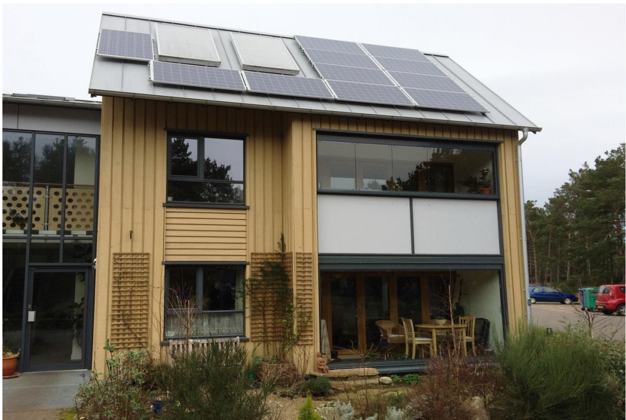
Photo: Eco-housing at the East Whins development at Findhorn include mechanical ventilation systems with heat recovery. Underfloor heating is fed by an air source heat pump in connection with solar thermal panels. Power is supplied from Solar PV panels and wind turbines located on the Park.
